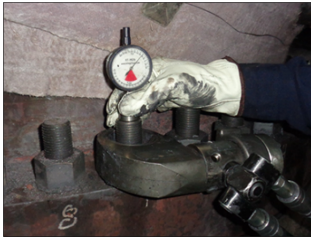
Bud Valve Torquing with RT-Bolt gauge
