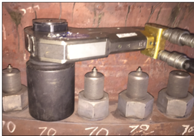
Torquing RT-Bolts with cassette type tool
